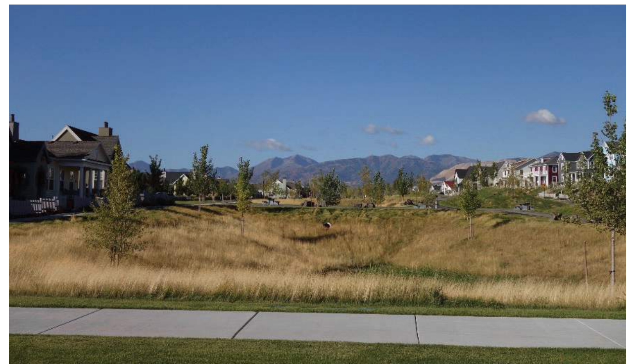
Stormwater basin planted with attractive native landscaping during a dry period
