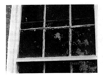
Note glazing putty breaking away from window pane frames. Former owners of the building installed storm windows, but damage to the existing windows has already progressed to point that all of the glazing putty will require replacement in the future if the widows are ever painted.
