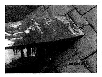
View of rusted/deteriorating metal parapet wall cap.
