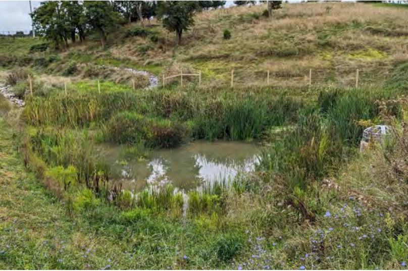
Stormwater BMP basin
