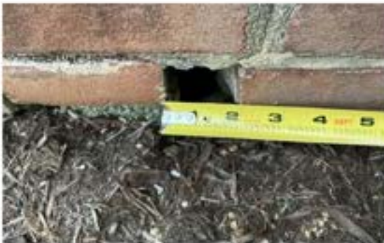
1" of forward movement has occurred at top step.
