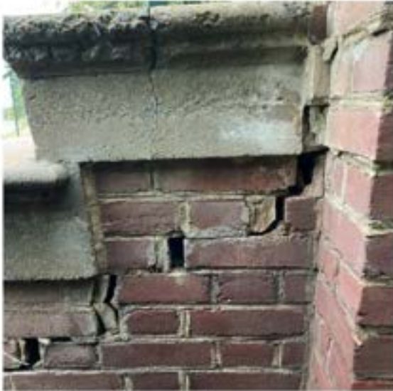
1" of forward movement has occurred at top step.
