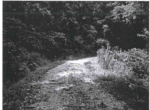
Picture of Easement, facing north
